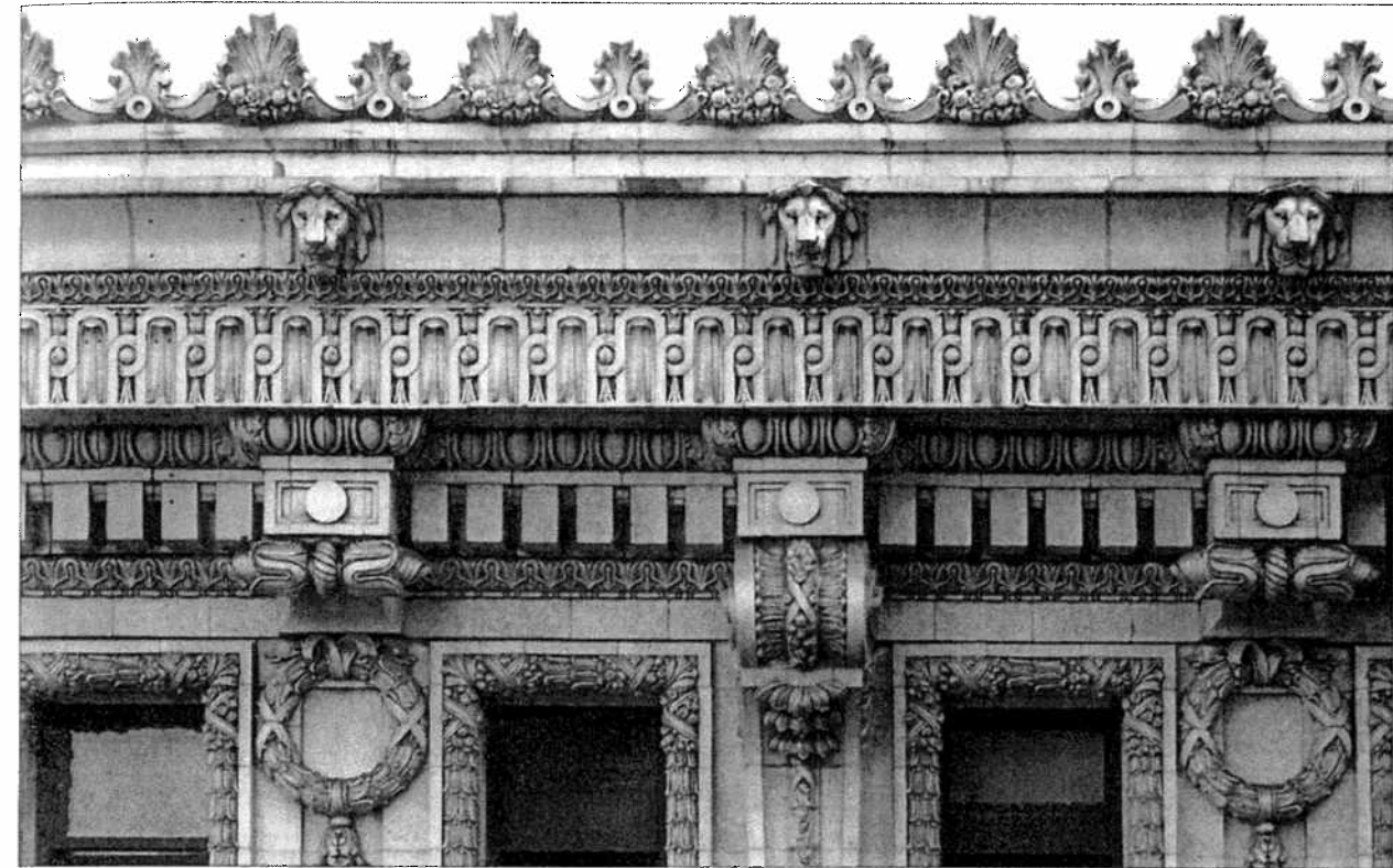
Above: The most elaborate terra cotta ornament of the building is on the cornice, with wreaths, dentils, multiple moldings, and lions' heads all surmounted by an anthemion crest.
